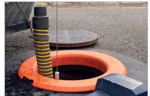
Sewer jet hose and camera protection
